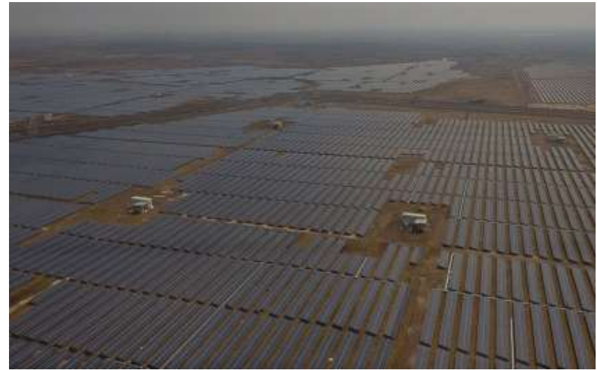
1000 MW solar park at Kurnool, AP, India
