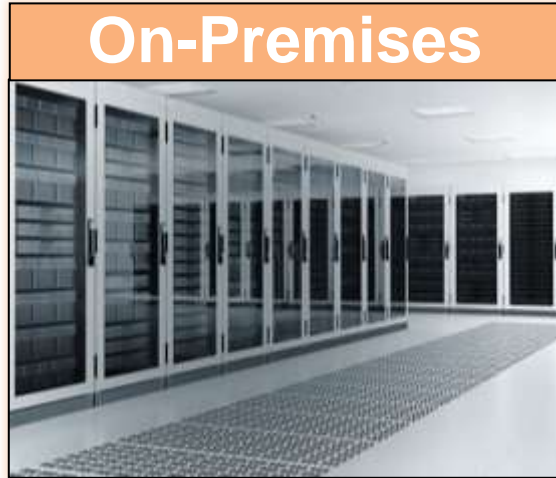
Data Center: Hisar
