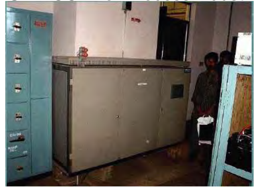
STATCOM for Process industries
