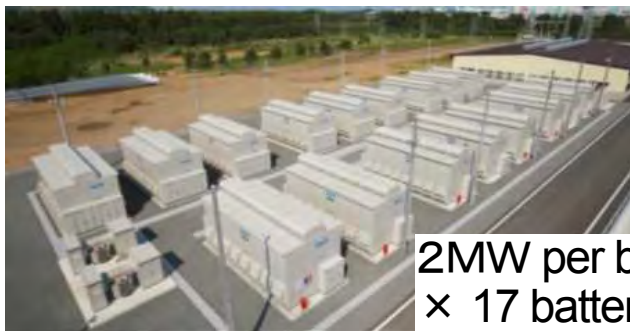
NAS Energy Storage System 34MW/224MWh (Operation started from 2008)
